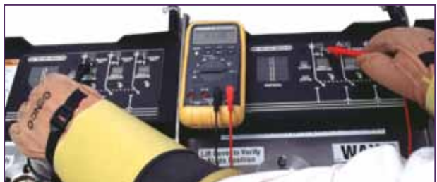
Figure 7. Measuring phase-to-phase voltage—Phase 1 to Phase 1.
