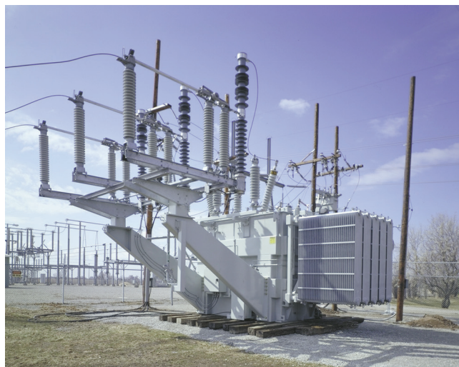
138-kV Trans-Rupter II Transformer Protector Model SE mounted to transformer at a temporary installation on railroad ties.
