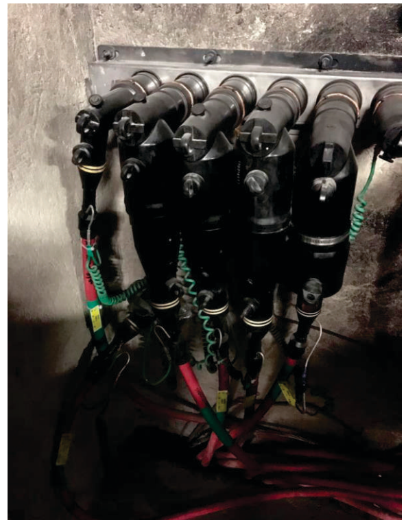
This application shows a Chardon MultiPoint Junction with Chardon Fused Elbows next to a competitor's Fused Elbow.
